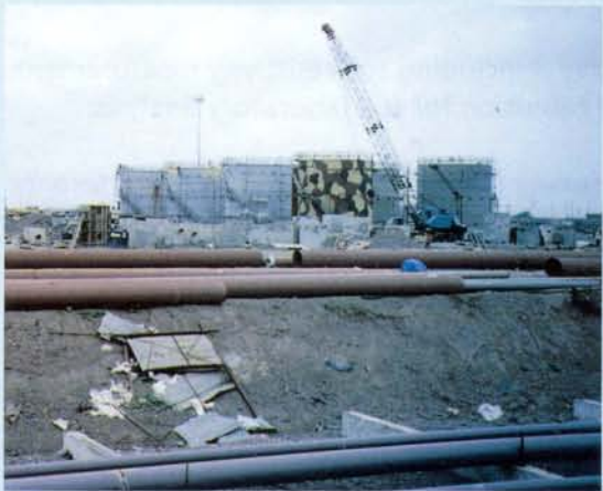
Corrpro Tank Grid CP Systems were installed on all tank bases at Reliance, Jamnager
