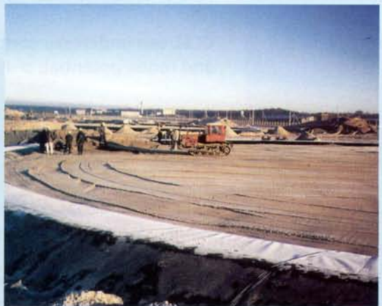
Tank base Cathodic Protection system installation
